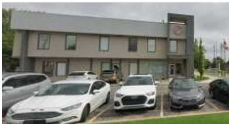
South side of building
